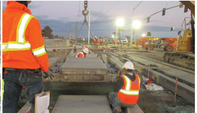
Crews install precast concrete panels at rail crossings.
